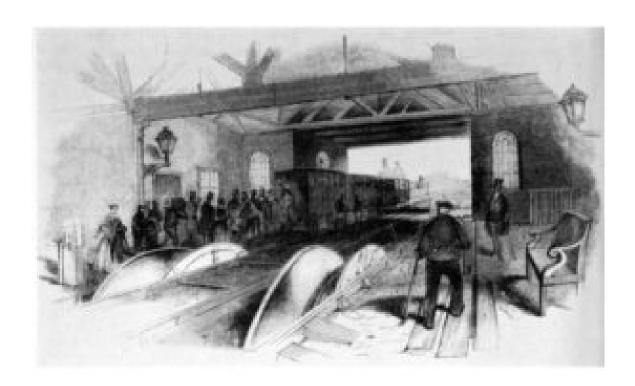
The Terminus at Minories c.1840 – note the engine-less carriages, the winding gear, the brakesman and, to the left the electric telegraph machine.
