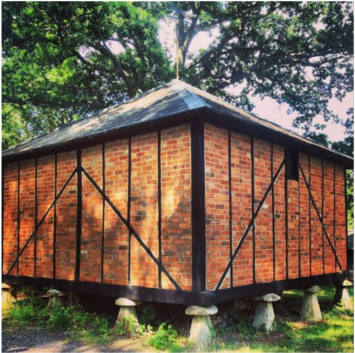
Above: Haversham Granary c.1835, raised on Staddle Stones. Now at The Chiltern Open Air Museum having been salvaged in 1991.[photo: A.Reeve]
