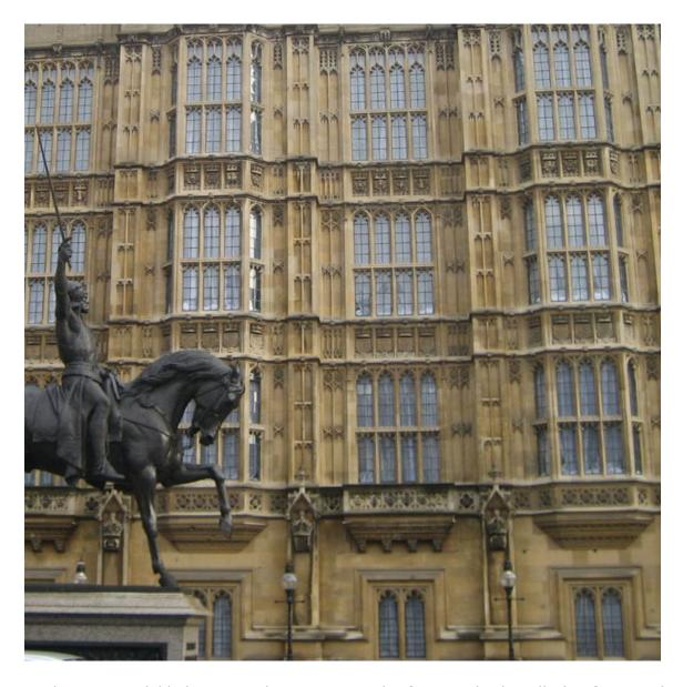
However, the stone quickly began to decay as a result of atmospheric pollution from coal burning in London and the poor quality of the material used. Although these defects in the choice of stone were visible as early as 1849, very little was done to prevent its decline during the 19th century. Barry himself experimented with various compositions on the stone and believed that the decay had been halted.
